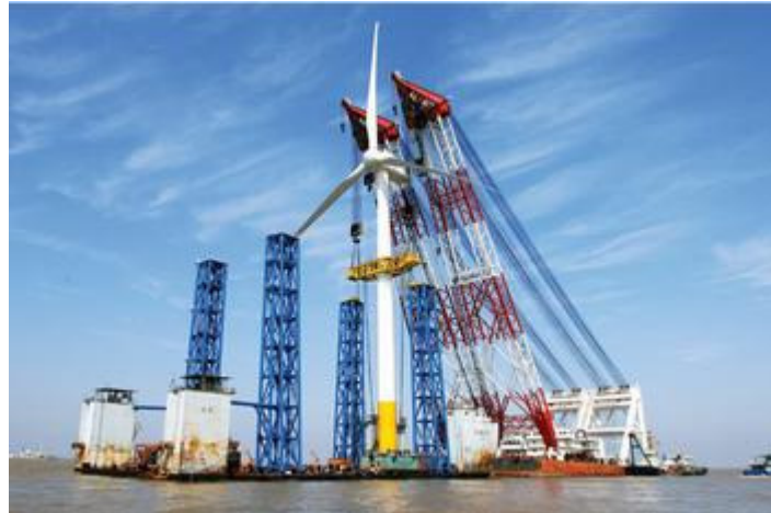
In February 2010, Beijing-based Sinovel Wind erected a 34th wind turbine close to Shanghai's Donghai Bridge. China's first offshore wind farm is capable of powering 200,000 households. (Photo by ANR2008)
