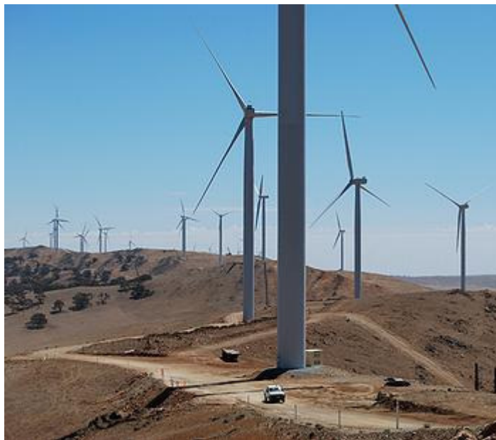
Hallett Wind Farm in South Australia, completed 2008 (Photo courtesy AGL Energy)
